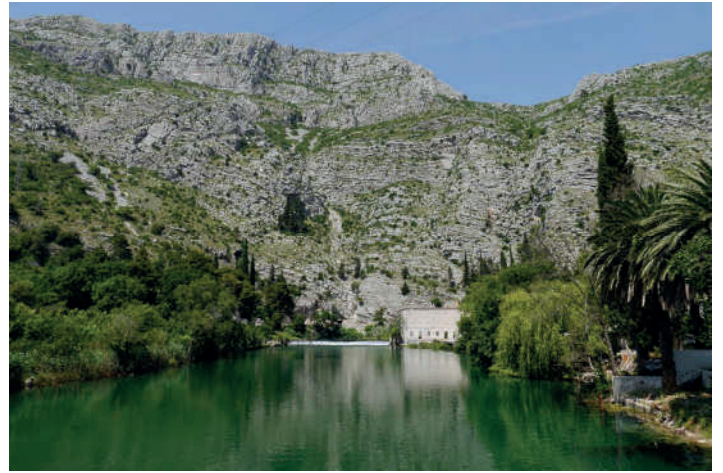
Ombla Spring, located on the Adriatic coast near Dubrovnik, Croatia, is one of the largest springs of the Dinaric karst region, with a minimum, mean and maximum discharge of about 4, 24 and 138 m 3 /s respectively. Originally, the spring discharged at sea level, but a small dam (2.4 m high) was constructed 50 m downstream of the spring orifice to avoid seawater intrusion. The spring water is used for the freshwater supply of Dubrovnik since 1897. Ph. Nico Goldscheider
